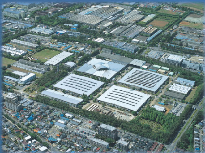
INDUSTRIAL COMPONENT & EQUIPMENT DIVISION
